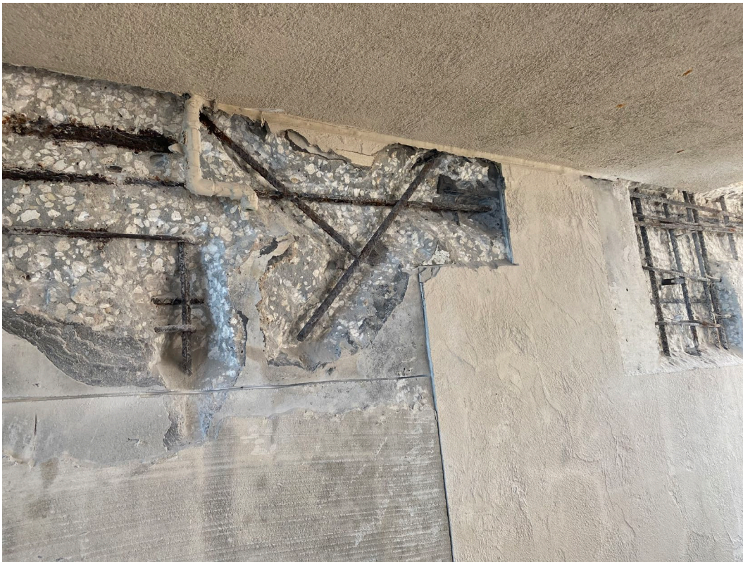
Picture 2: In-progress concrete repairs
