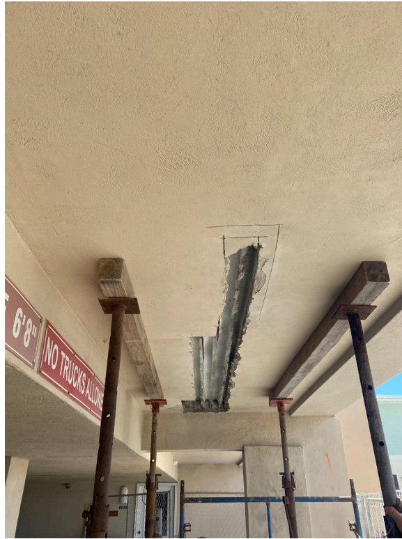
Picture 3: In-progress slab repair below 1 st floor walkway
