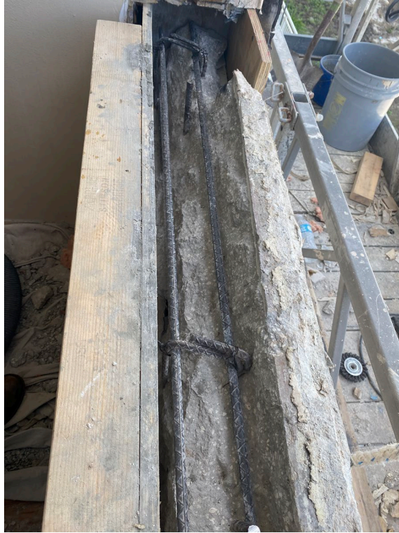
Picture 1: Unit 208 window sill repair
